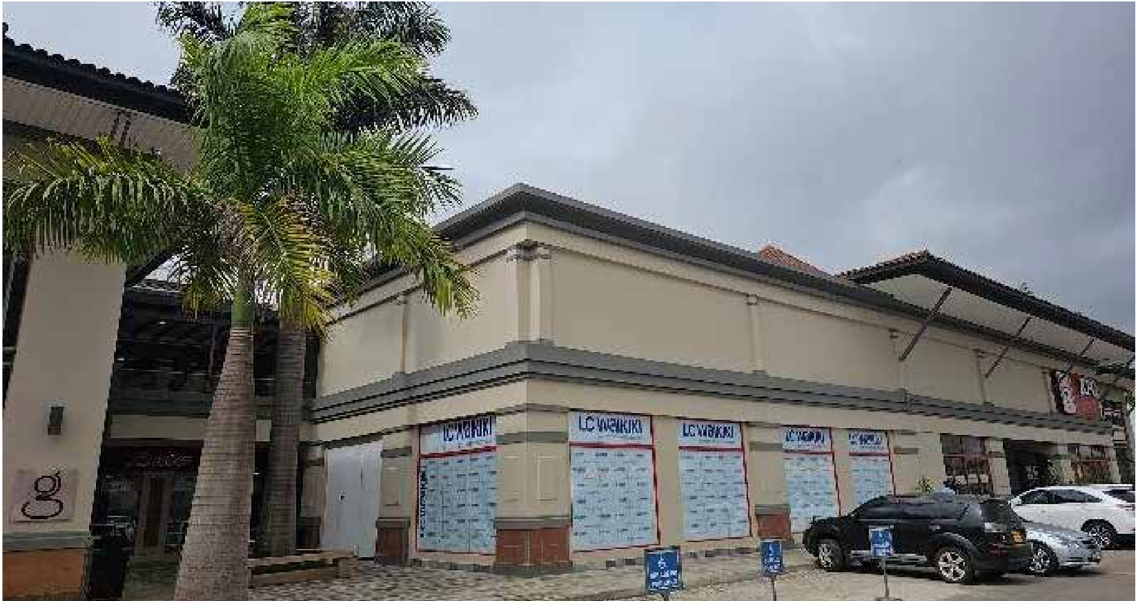
LC Waikiki Retail Store Galleria Mall
