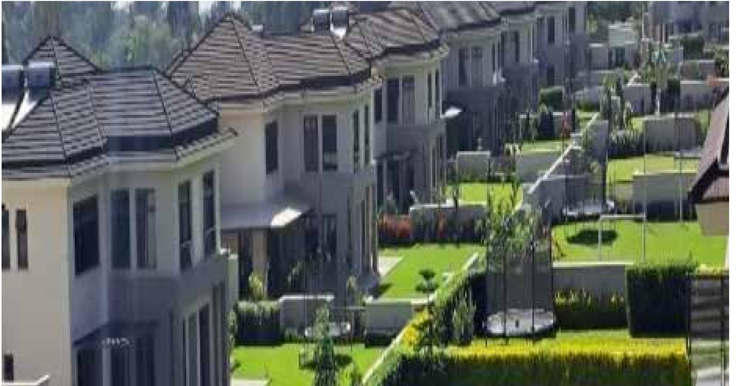
GALLERIA GARDENS PHASE II on plot LR NO. 2248/6
